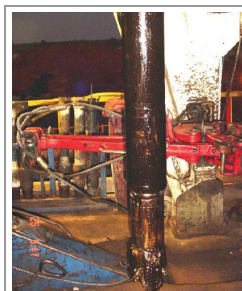
Oil coating 6-inch drill bit during horizontal drilling operations
